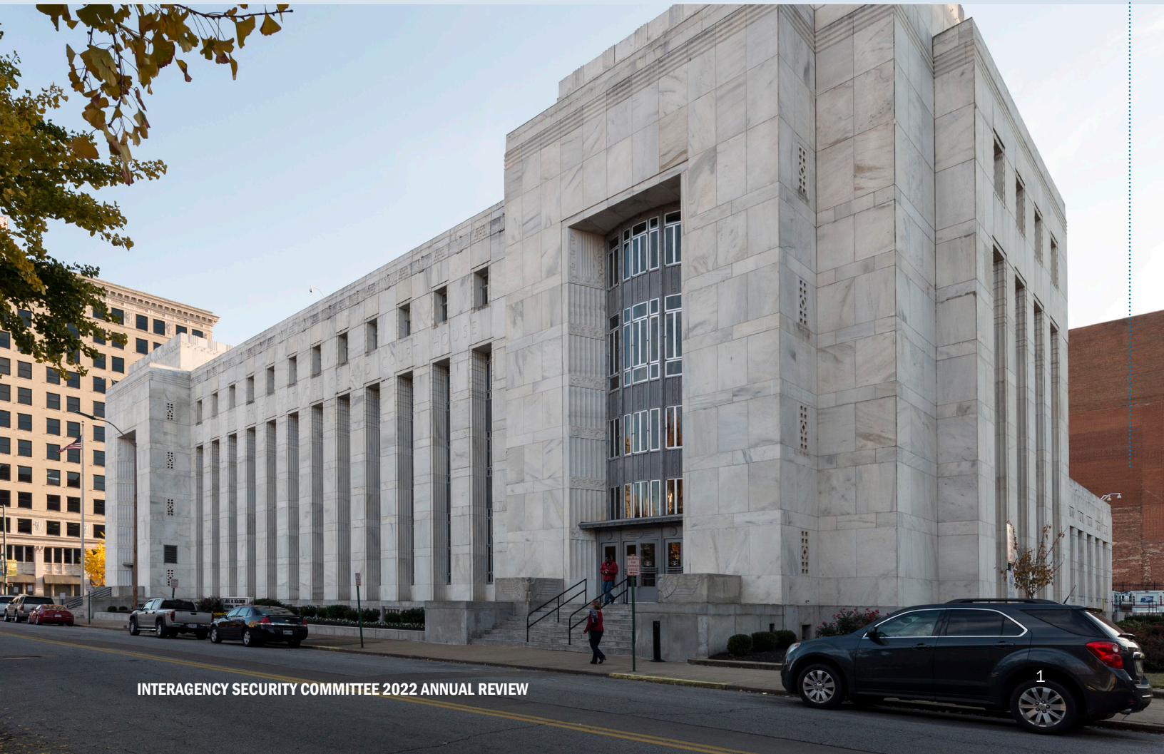
Below: The Joel Solomon Federal Building and U.S. Courthouse, Chattanooga, TN Previous: Ewing T. Kerr Federal Building, Casper, WY Credit: U.S. General Services Administration Historic Building Photographs
