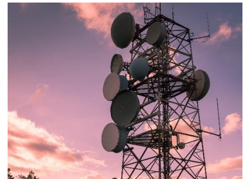
Image of a Radio Communications Tower
