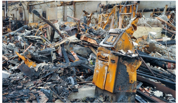
Source: FEMA Photo Library
