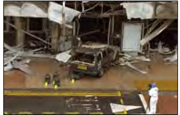
Figure 12: Glasgow International Airport Incident (2007) Property of DHS
