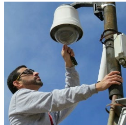
An employee checks a camera is working properly. (Source: DOS)
