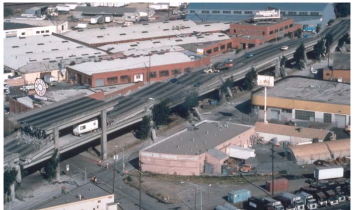
Damage to Interstate 880 in Loma Prieta earthquake, Oct. 1989 (Creative Commons/Joe Lewis)
