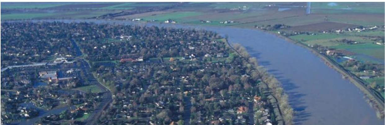
Levees along a riverbank (Source: DHS)
